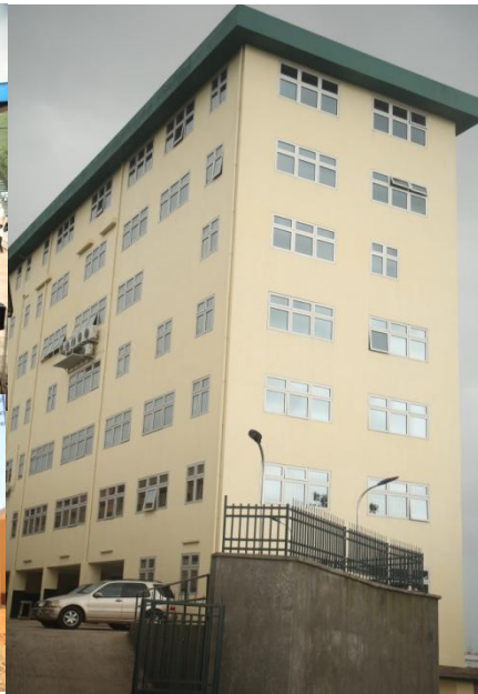
Newly constructed Ekundayo Thompson Building- IPAM, Tower Hill
